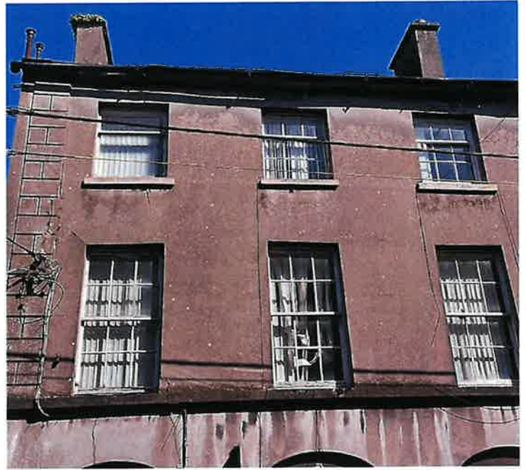
Above: Images H & I front façade showing crack above entrance doorway, staining and untidy wiring & to the right, shows windows with damaged timber and paintwork.
