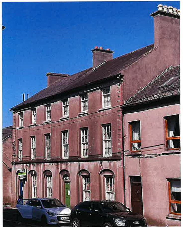
Above: Images J & K showing front façade cracked and stained, roof eaves and gutter in poor / rotting condition, first floor windows damaged / broken sashes & showing curtains / blinds discoloured and in poor condition, taken from the site visit 30 th April 2025.
