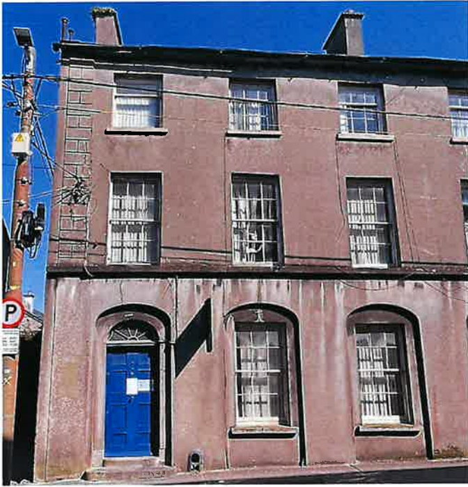
Above: Images H & I front façade showing crack above entrance doorway, staining and untidy wiring & to the right, shows windows with damaged timber and paintwork.
