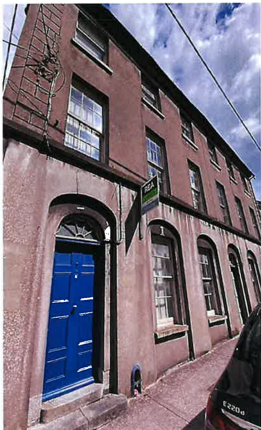
Images A & B above and images C & D below, from November 2023: Front view of the property from Church St. showing broken / damaged windows, peeling paintwork to timber windows and main doorway, and poor condition / stained appearance of the front and gable façade of the building, and the rear and side of the property onto Bath St heavily overgrown with vegetation.
