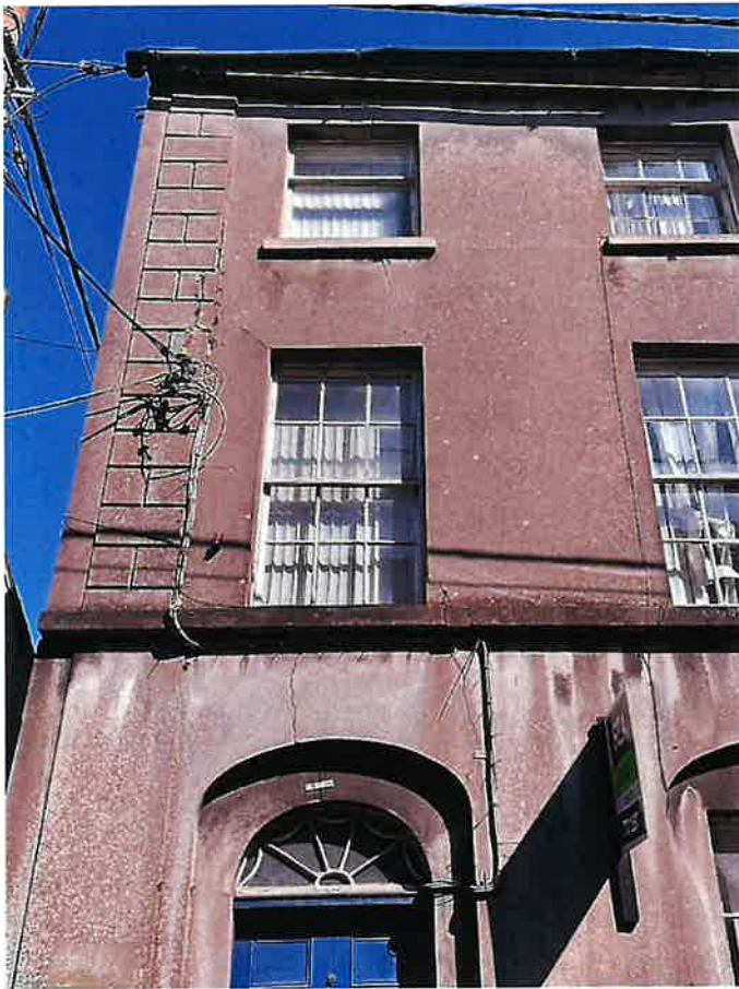
Above: Images J & K showing front façade cracked and stained, roof eaves and gutter in poor / rotting condition, first floor windows damaged / broken sashes & showing curtains / blinds discoloured and in poor condition, taken from the site visit 30 th April 2025.
