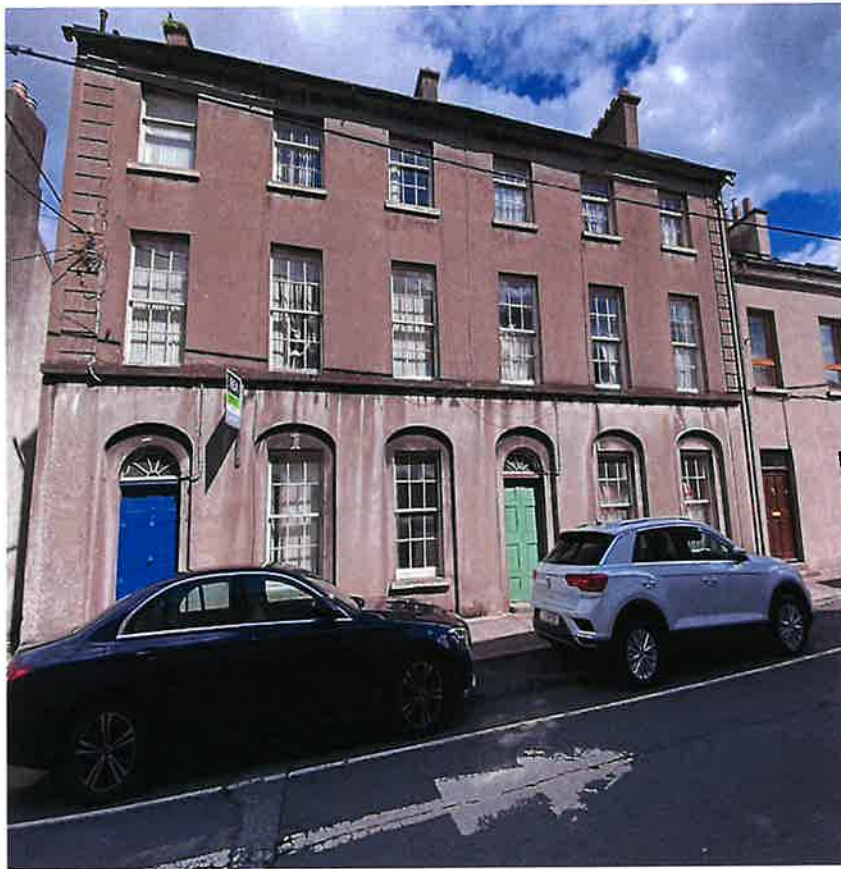
Images A & B above and images C & D below, from November 2023: Front view of the property from Church St. showing broken / damaged windows, peeling paintwork to timber windows and main doorway, and poor condition / stained appearance of the front and gable façade of the building, and the rear and side of the property onto Bath St heavily overgrown with vegetation.
