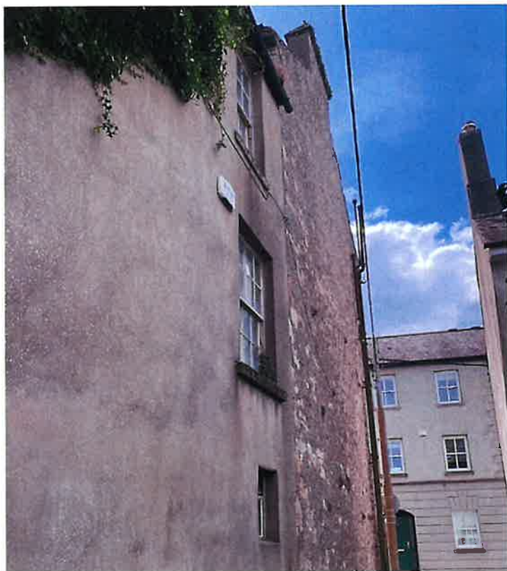
Images A & B above and images C & D below, from November 2023: Front view of the property from Church St. showing broken / damaged windows, peeling paintwork to timber windows and main doorway, and poor condition / stained appearance of the front and gable façade of the building, and the rear and side of the property onto Bath St heavily overgrown with vegetation.
