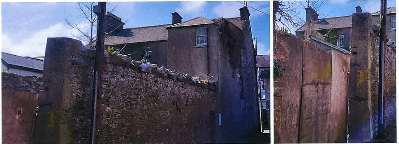
Above: Images F & G from 1 st April 2025, showing rear upper windows of 21 Church St. in broken / damaged condition, vegetation growing from the roof / gutter and along the side gable. Rear roof gutter and downpipe look in poor condition also.
